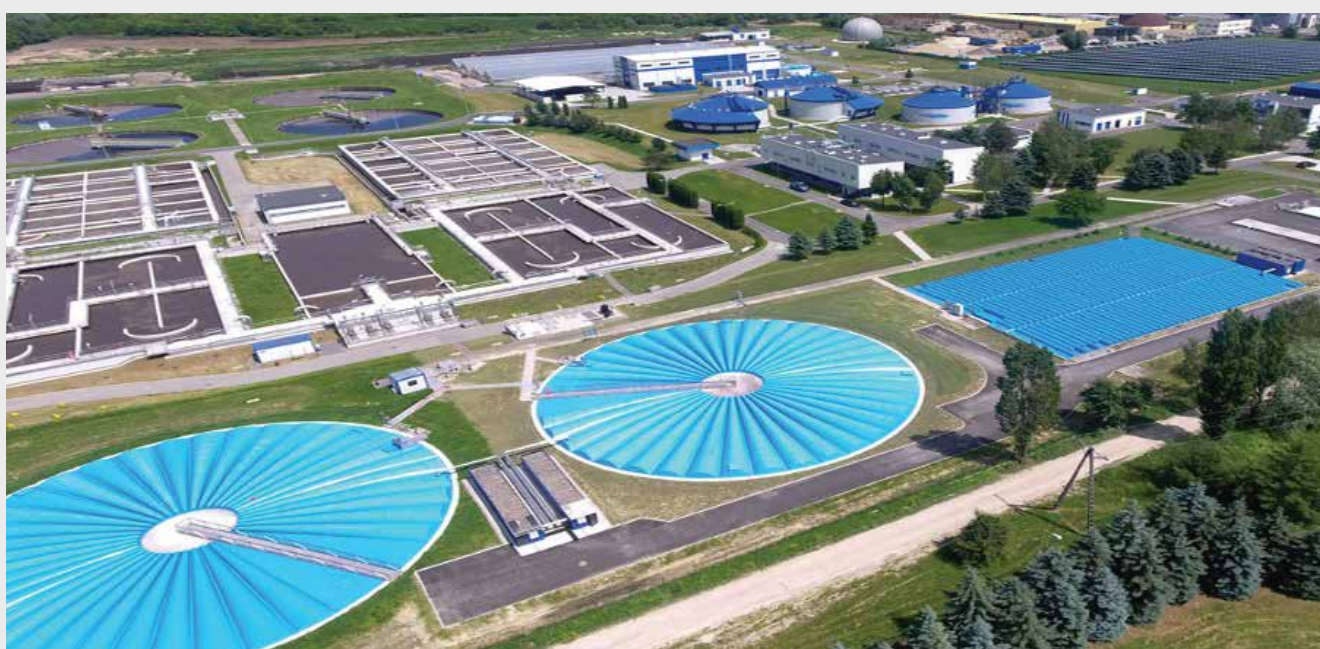
Figure 1. Aerial, Rzeszow WWTP.
