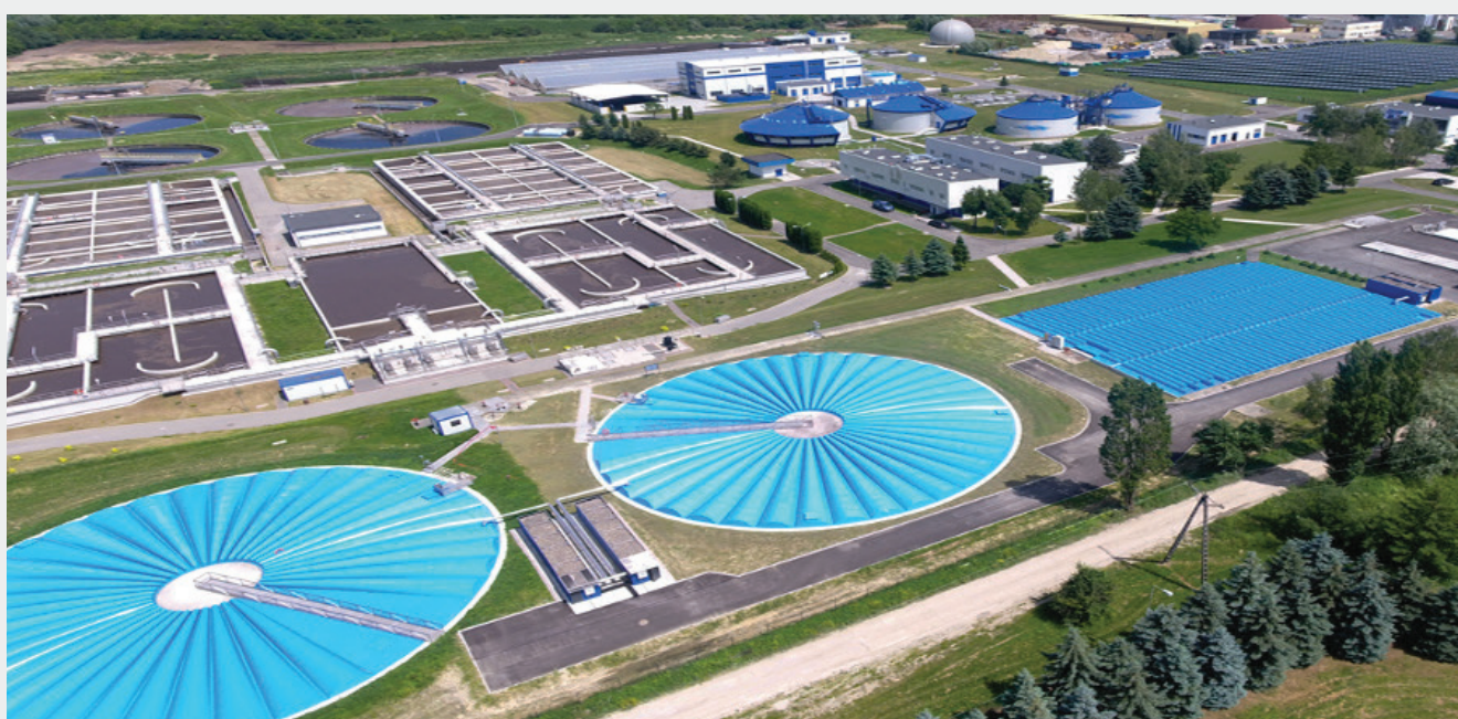
Figure 1. Aerial, Rzeszow WWTP.
