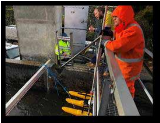
Image 7. Monpeelyata Canal gauging bridge. This image shows ADCP and CM being deployed simultaneously. CM measurements are made using a canal rod, and ADCP measurements by sliding its securing line along the canal's structural pier to the appropriate chainage.
