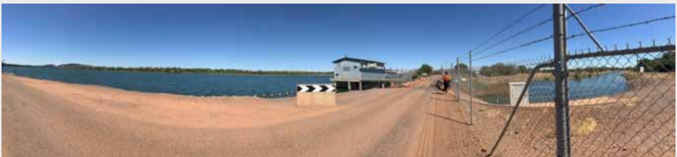
Figure 1. Lake Kununurra to M1 Irrigation Channel (decommissioned Pump Station in the Centre) left to right. (Right Bank viewing DS).
