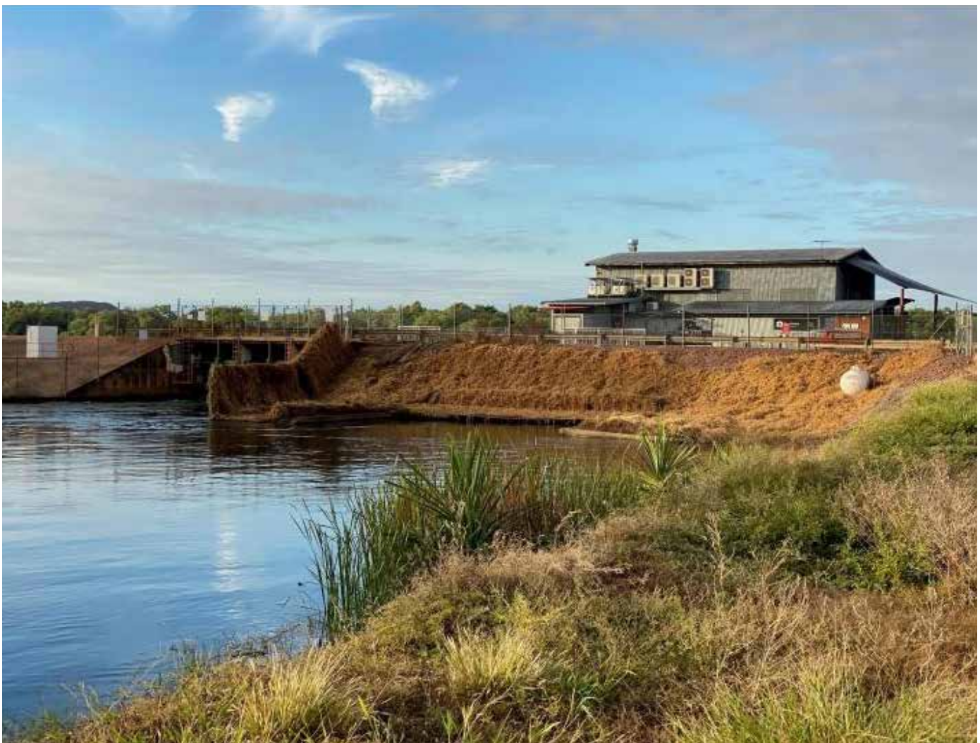
Figure 4. M1 Intake Radial Gates (left) and Pump Station (Right) as taken at the old M1 Gauging Station Hut (Looking US).
