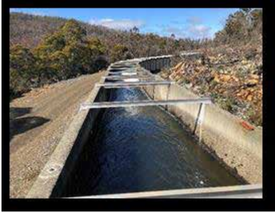
Images 5 & 6. Monpeelyata Canal upstream approach and downstream departure. Note the presence of the hydraulic jump downstream of the gauging station in image 6.
