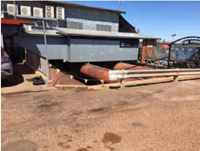
Figure 2. Heritage Listed Pump House.
