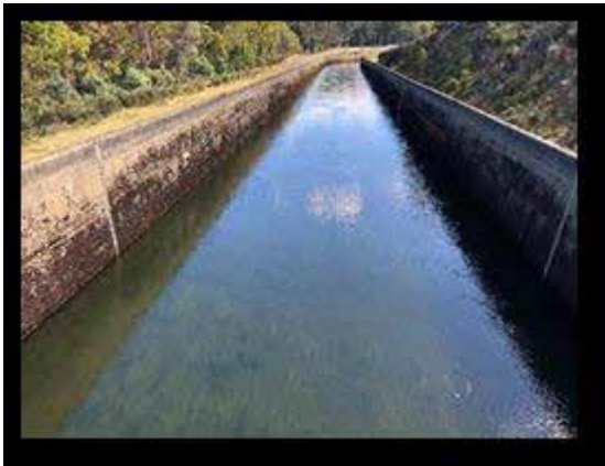
Images 1 & 2. Bronte Canal upstream approach and downstream departure. Note shallower conditions within image 1 demonstrating the presence of algae lining the bottom of the canal.
