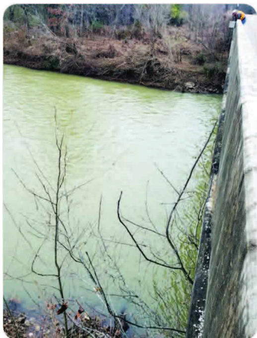
Figure 16. USGS gauging station 07048600 on the White River near Fayetteville, AR (USA). Photo and data courtesy of Neil Holaway, USGS.
