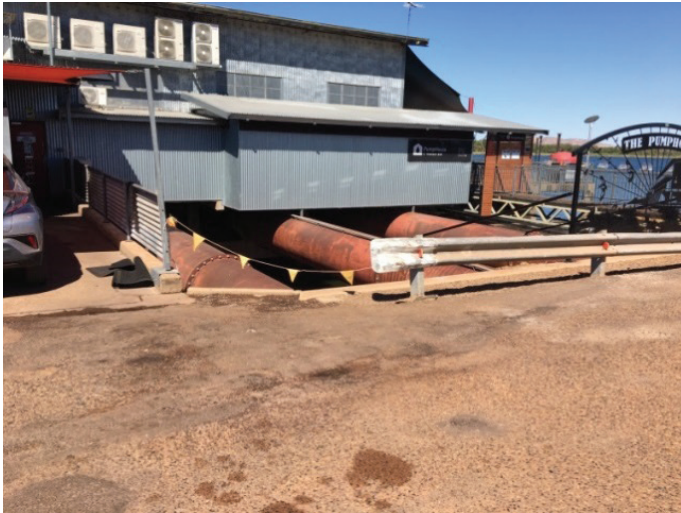
Figure 2. Heritage Listed Pump House.
