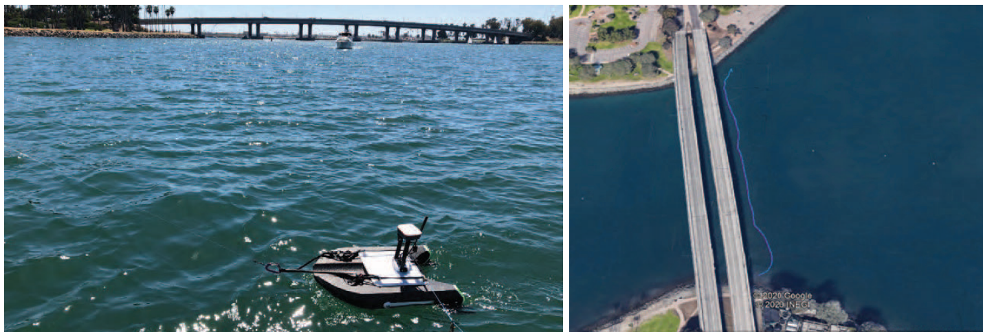
Figure 20. Bridge and transect path upstream of bridge.
