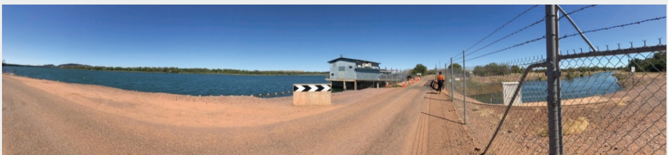
Figure 1. Lake Kununurra to M1 Irrigation Channel (decommissioned Pump Station in the Centre) left to right. (Right Bank viewing DS).
