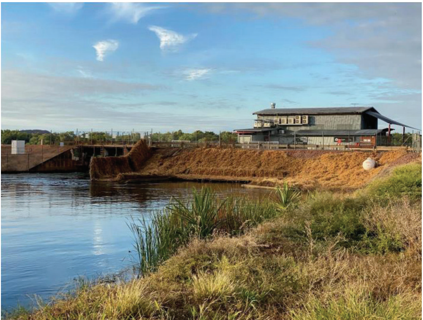
Figure 4. M1 Intake Radial Gates (left) and Pump Station (Right) as taken at the old M1 Gauging Station Hut (Looking US).
