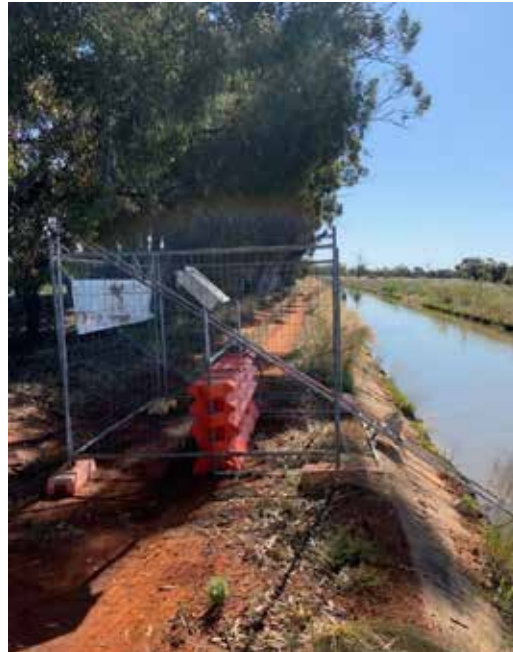
Figure 5. Temporary ADVM mounting frame.
