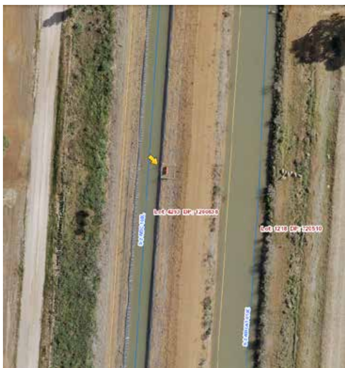
Figure 2. Aerial view of SL1500-3G site installation on the NBC.
