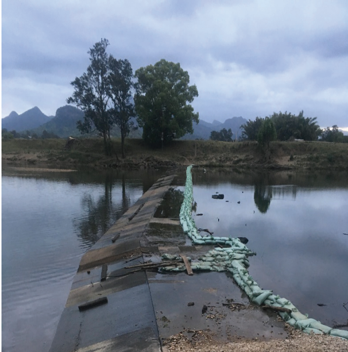
Figure 8. Tweed Shire Councils overtopping prevention controls using sandbags and concrete blocks (Source: Tweed Shire Council).
