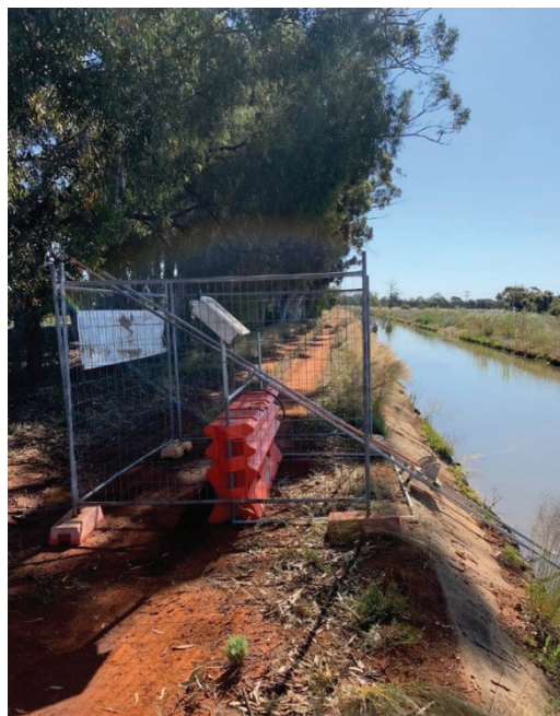
Figure 5. Temporary ADVM mounting frame.
