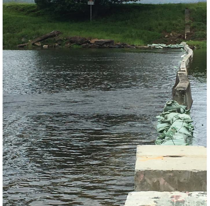
Figure 8. Tweed Shire Councils overtopping prevention controls using sandbags and concrete blocks (Source: Tweed Shire Council).
