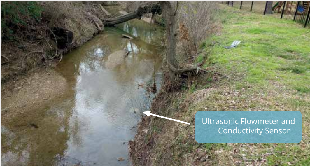
Figure 1. Cottonwood Creek installation.
