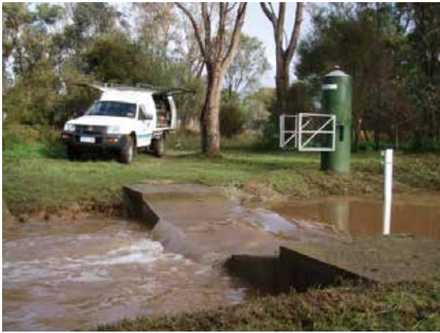
Figure 2. 609020 Walker Rd Gauging Station, Narrogin.
