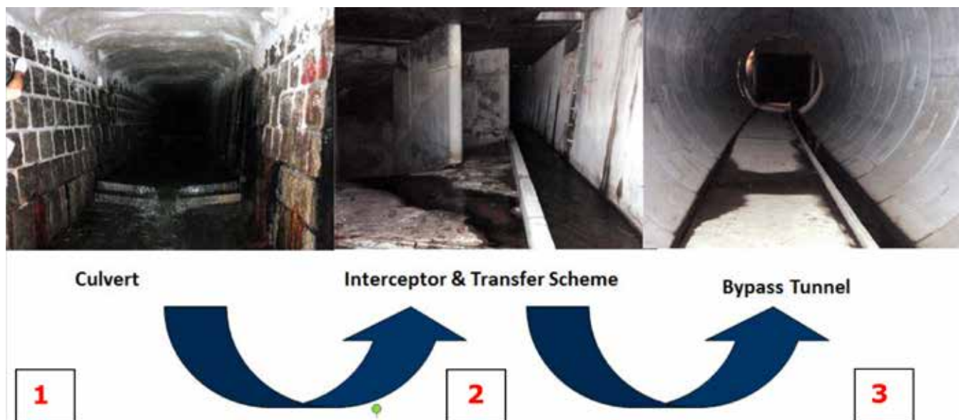
Figure 6. Interceptor Schematic.
