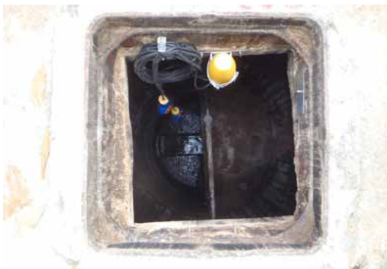
Figure 2. High Water Level Alarm System installed in Manhole
