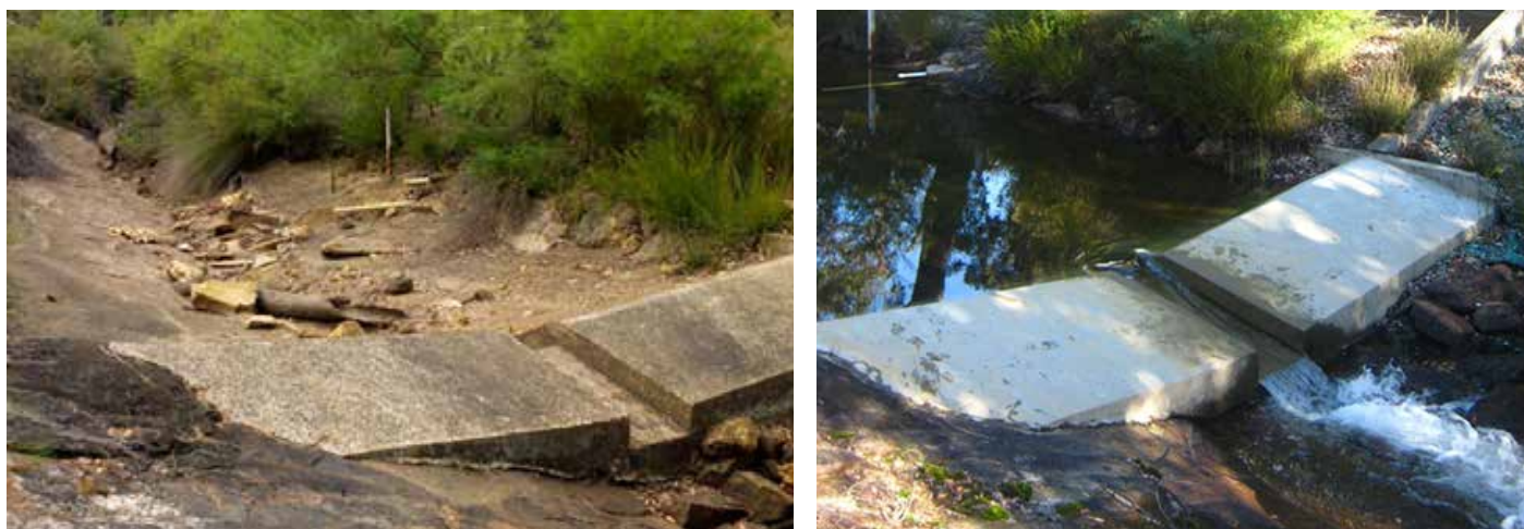
Figure 5. Vardi Rd Gauging Station Weir prior and post resurfacing.
