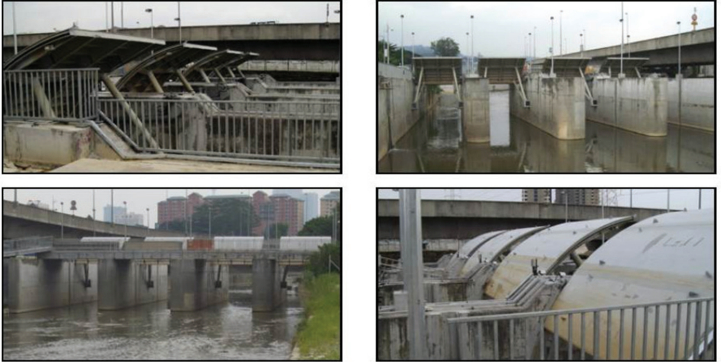
Figure 2. Radial Undershot Gates, controlled by the Flood Detection System, regulate flow to the City and into the tunnel.
