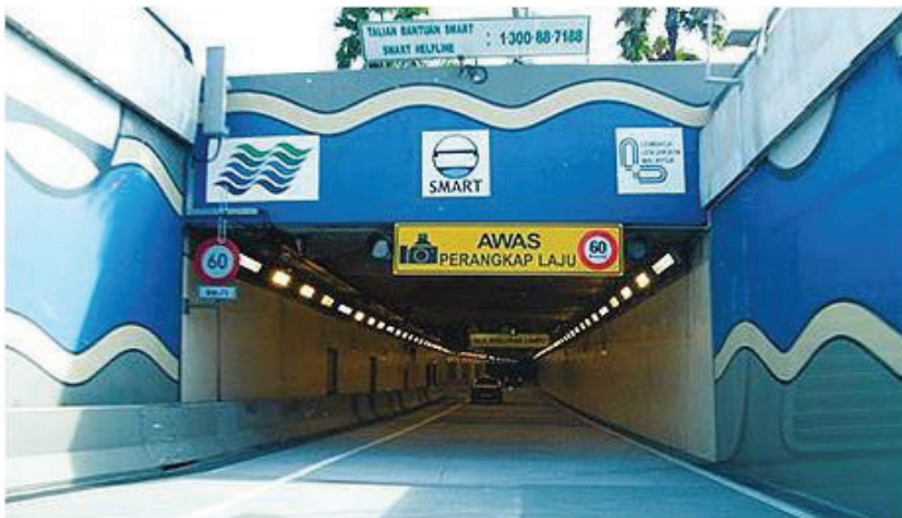
Figure 5. Entrance to the SMART Tunnel upper traffic deck.
