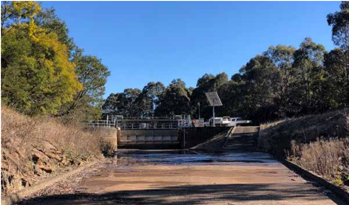
Figure 5: Upstream, looking downstream towards radial gate.
