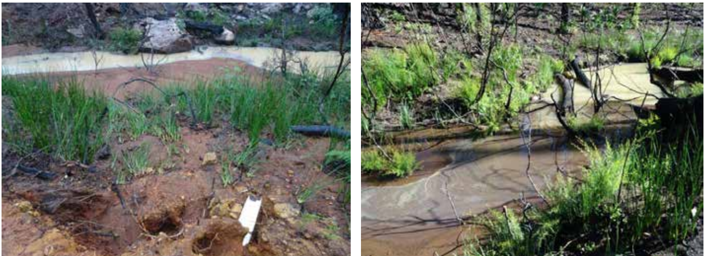
Figure 13: Samson Dam to Pipehead Creek Line. Left: Bank erosion, Right: Suspended sediments in the brook, post rainfall event May 2016 (Images by M. Sturges, Arrona 2016).
