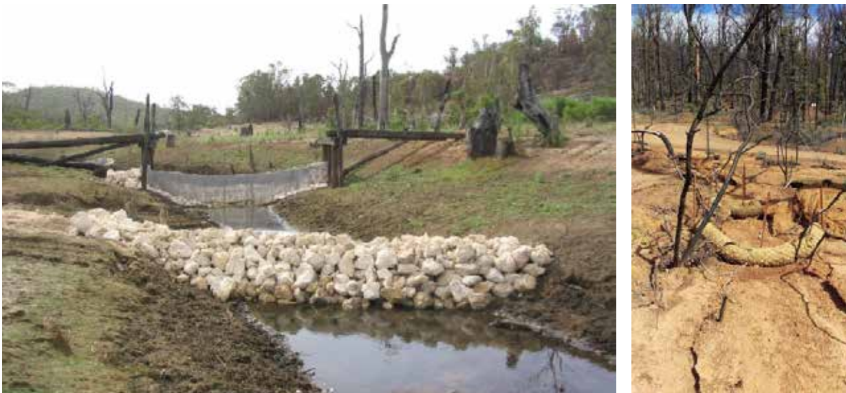
Figure 21: Left: limestone and geofabric sedimentation structures installed in Mundaring Catchment post 2005 Hills fire, Right: Coir Logs installed near 6215W000 Samson Brook at Scarp Rd.
