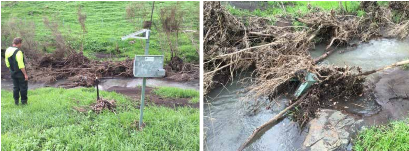
Figure 16: Damage to 6215W002 Samson Brook at Paddock East June 2016 (4 months after the fire).
