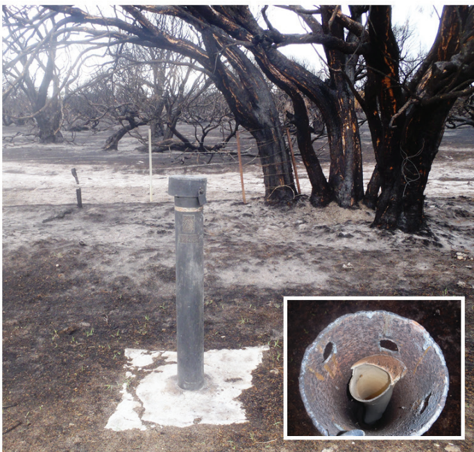
Figure 5: Bore HS24A, Damage to surrounds and inner casing post Waroona Fire.
