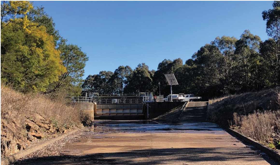
Figure 5: Upstream, looking downstream towards radial gate.
