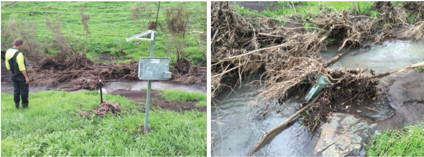
Figure 16: Damage to 6215W002 Samson Brook at Paddock East June 2016 (4 months after the fire).
