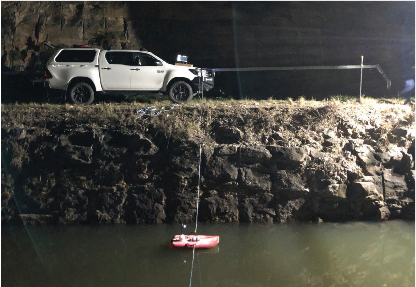
Figure 14: Equipment setup in preparation for pump run measurement.
