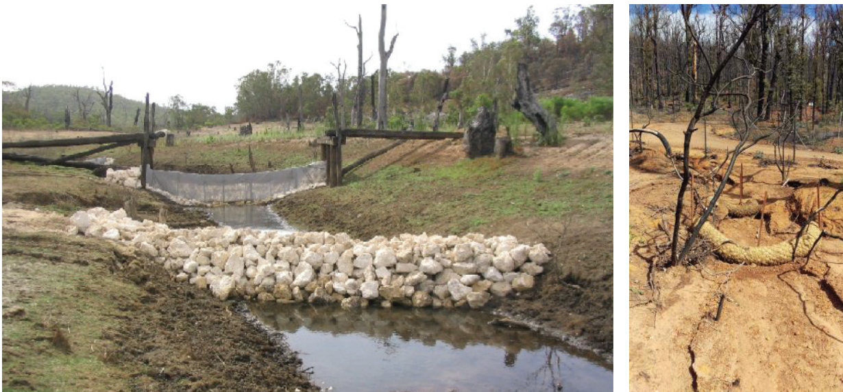
Figure 21: Left: limestone and geofabric sedimentation structures installed in Mundaring Catchment post 2005 Hills fire, Right: Coir Logs installed near 6215W000 Samson Brook at Scarp Rd.
