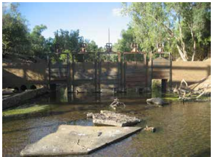
Figure 7: Offtake Gates to Uralla Creek.
