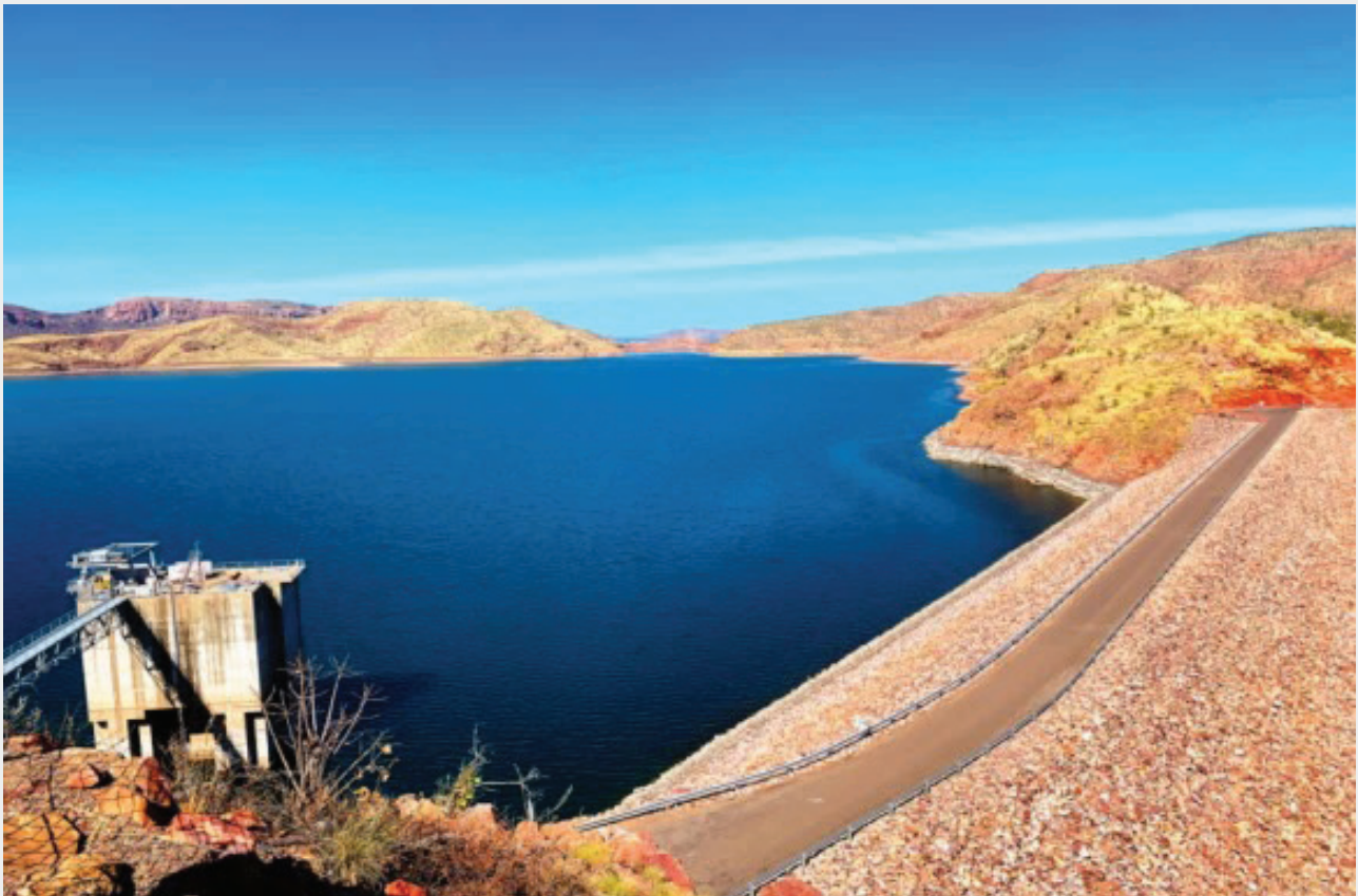
Figure 1: Ord Dam and (a small part of) Lake Argyle.
