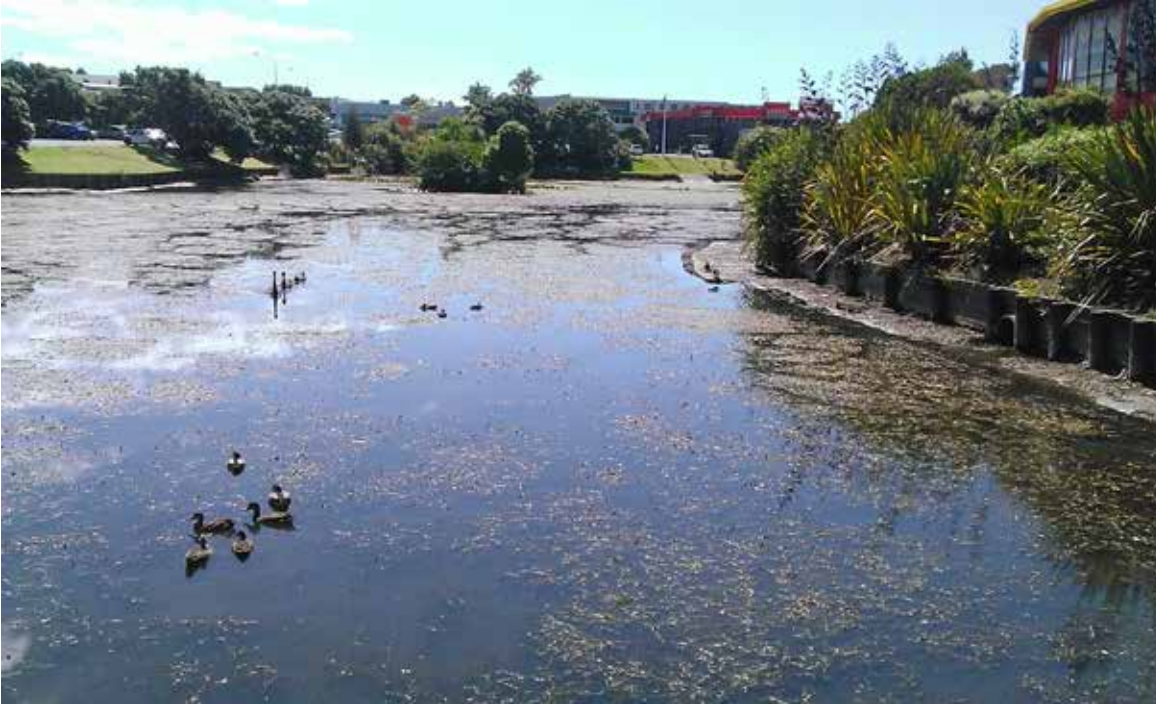
Figure 4: Auckland stormwater pond with extensive weed growth.
