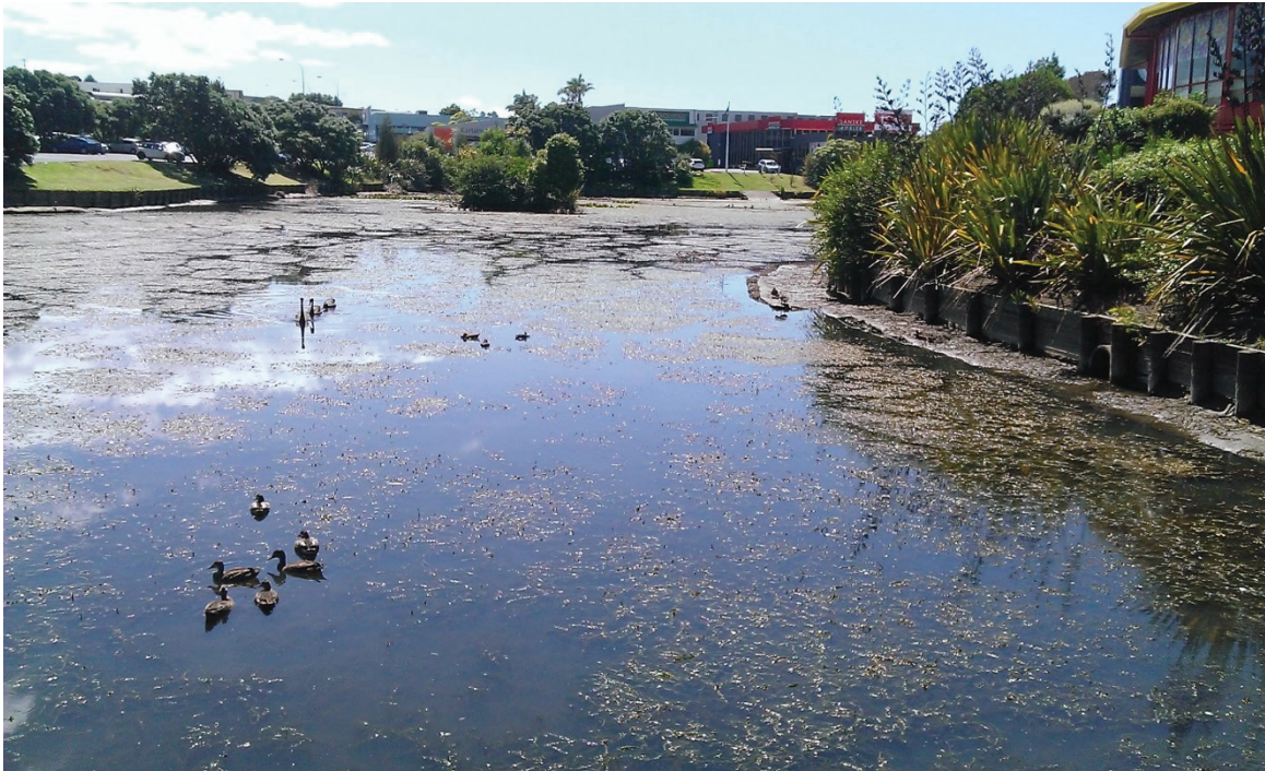
Figure 4: Auckland stormwater pond with extensive weed growth.
