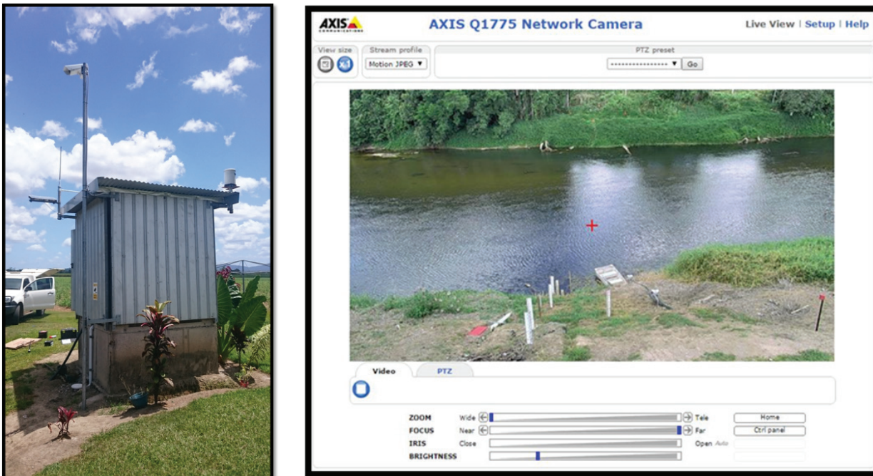
Figure 4. An example of an in-situ camera installation and its view of the river. Located at GS111101D Russel River at Bucklands.
