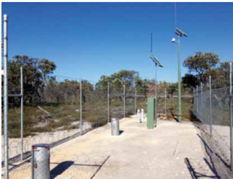
NG3 IP Telemetry site with IP Camera.
