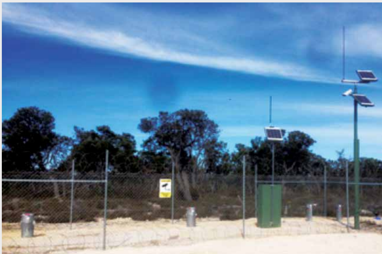
Upgrade solar panel array installed.
