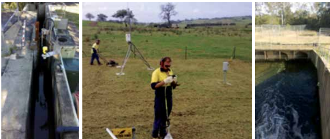
Figure 10. Images of hydrometric monitoring stations at WWTP and WRP. The left image shows Riverstone influent monitoring station where a level sensor and a flume structure are used to calculate flows. The Middle image is at Gerroa weather station where rain, humidity, solar radiation, wind speed and direction are monitored. The right image is at St Mary's effluent monitoring station, where tertiary level treated wastewater is released into local waterways.
