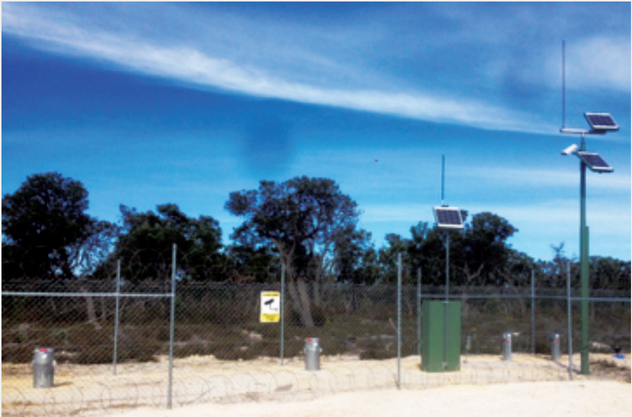
Upgrade solar panel array installed.
