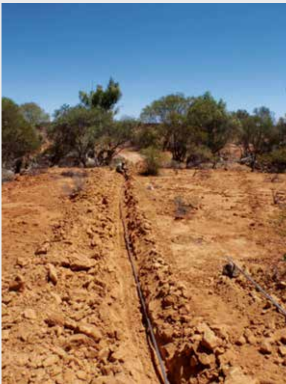
Installing the bubble line
