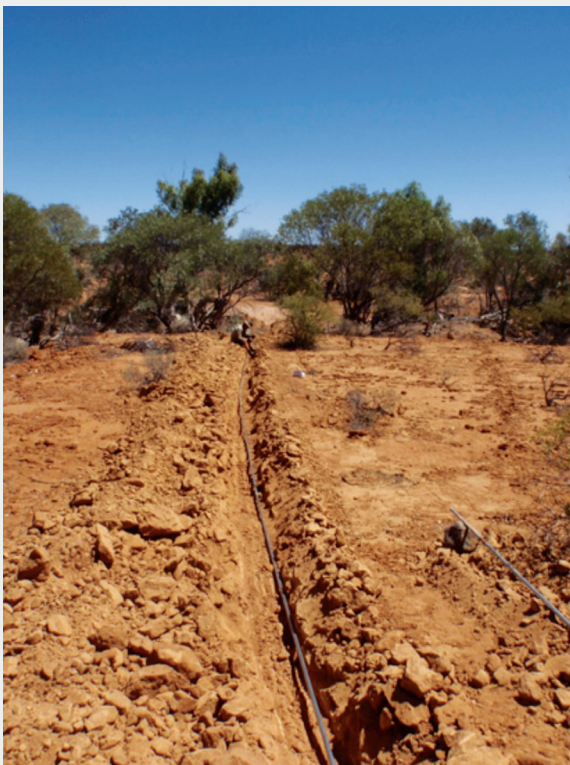
Installing the bubble line
