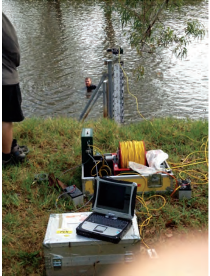
Bore hole camera being fed into inlet.
