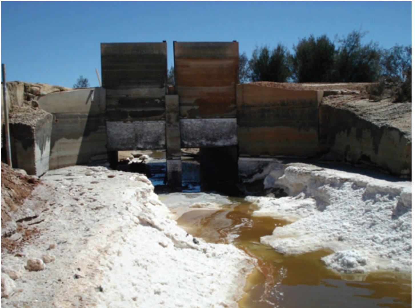
Gates (open in the picture) controlling water releases into the Avon River. (Yes, that's salt on the banks, and that is after much of it had been flushed away.)
