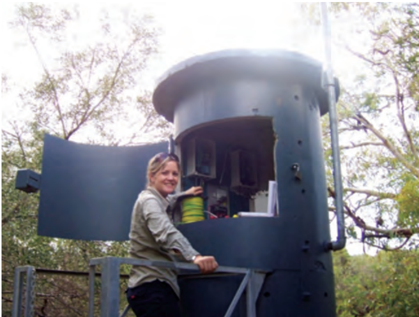
Hill River float well Neon install.
