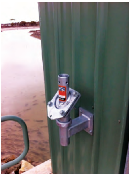
External swivel pole bracket / friction plate.
