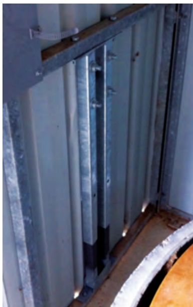
Internal adjustable wall bracket.
