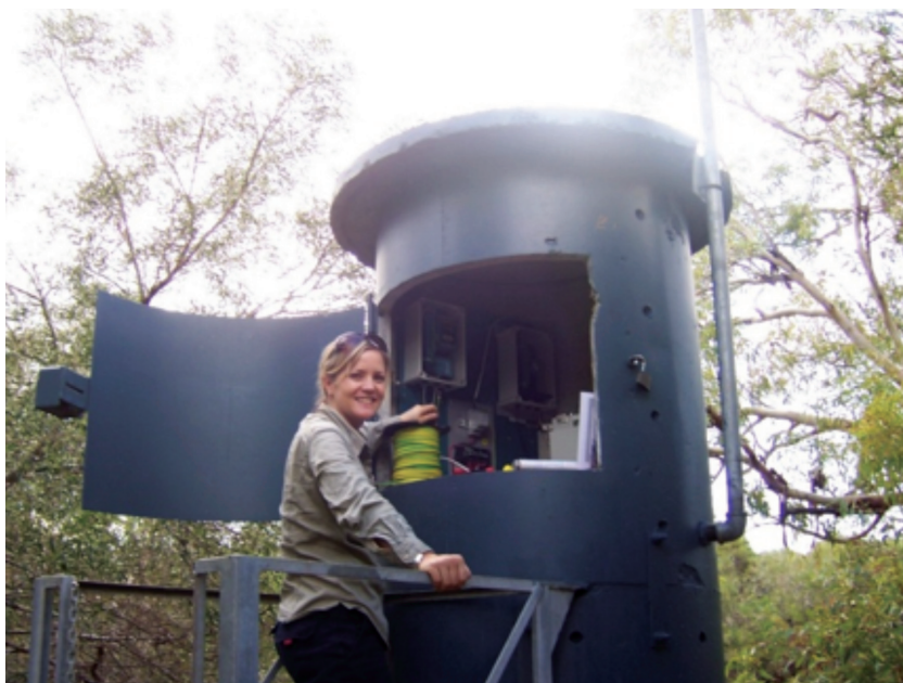
Hill River float well Neon install.
