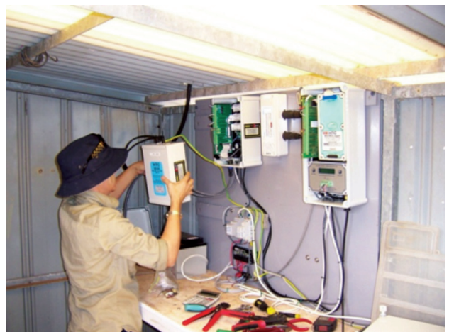
Another Neon install at Emu Springs.
