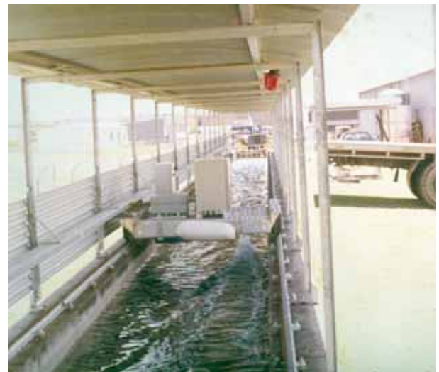
Upgraded Trolley and partially enclosed flume
