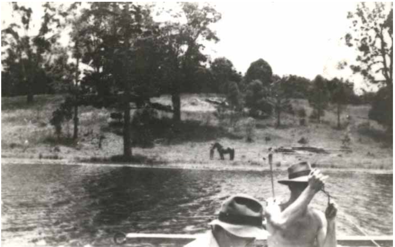
RATING METERS ENOGGERA RESERVOIR 1949
