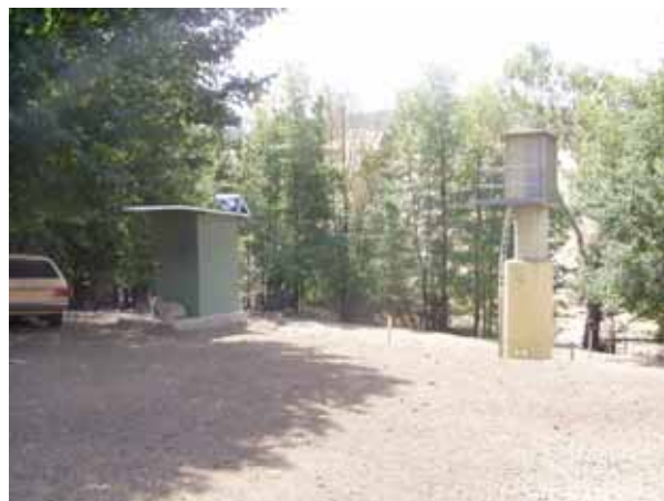
Photograph 5 - Upgraded site now at ground level (old structure to be removed).
