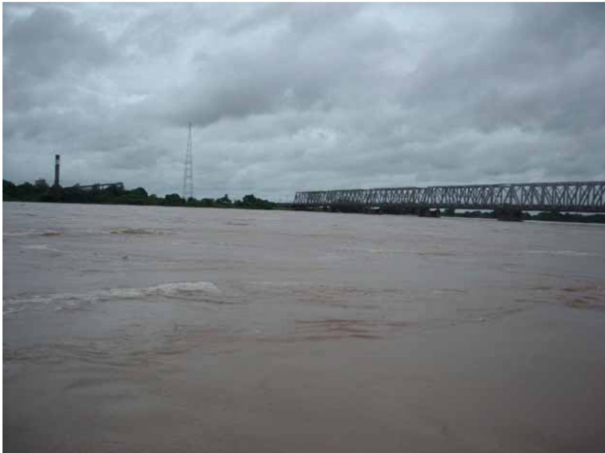
120001A Inkerman Bridge, Sugar Mill on right bank
