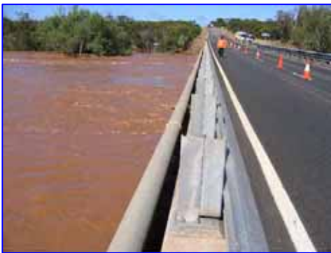
Traffic controllers at Eradu
