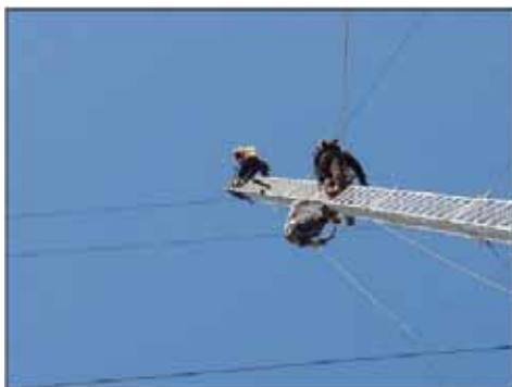
Figure 3.1 Monitoring Tower Construction
