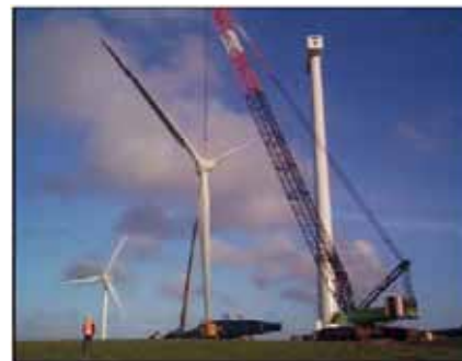
Figure 1.1 Woolnorth Wind Farm Construction
