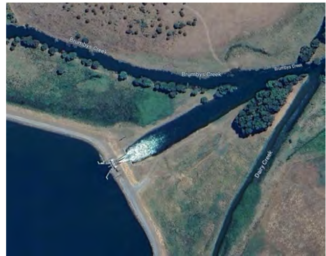
Figure 2. Outflow Stretch from Regulating Structure
